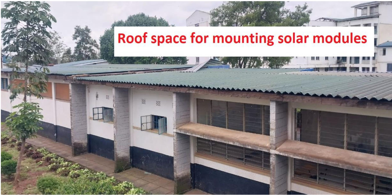
Figure 5: PV installation roof
