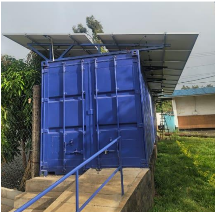
Figure 4: Existing 11.7kW PV system and LV AC panel (about 20 metres from the machine room of the proposed captive solar generation system)
