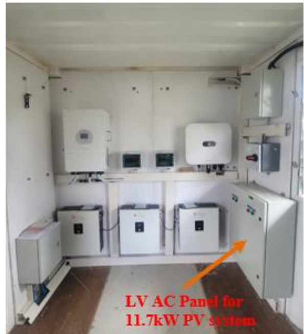
Figure 4: Existing 11.7kW PV system and LV AC panel (about 20 metres from the machine room of the proposed captive solar generation system)
